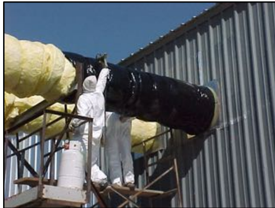
Applying Cotton Koozie Shrink Wrap Film over fiberglass batt insulation.
