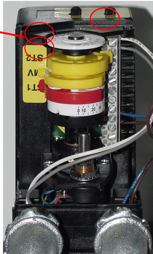
GVM Gas Valve Motor adjustment
