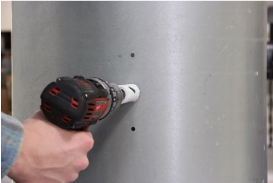
Figure 3: Cut out the middle hole
