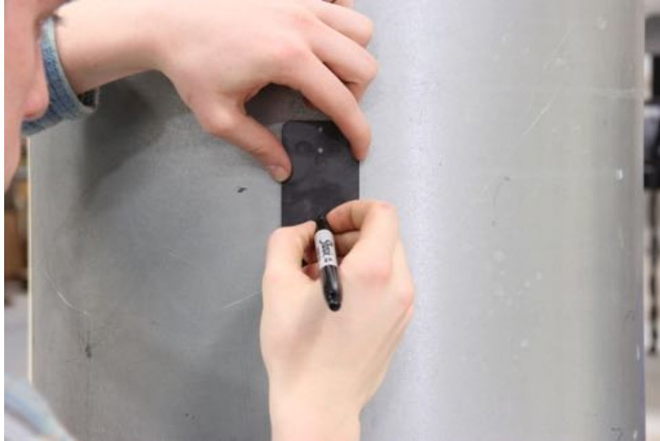
Figure 1: Mark the holes using the template
