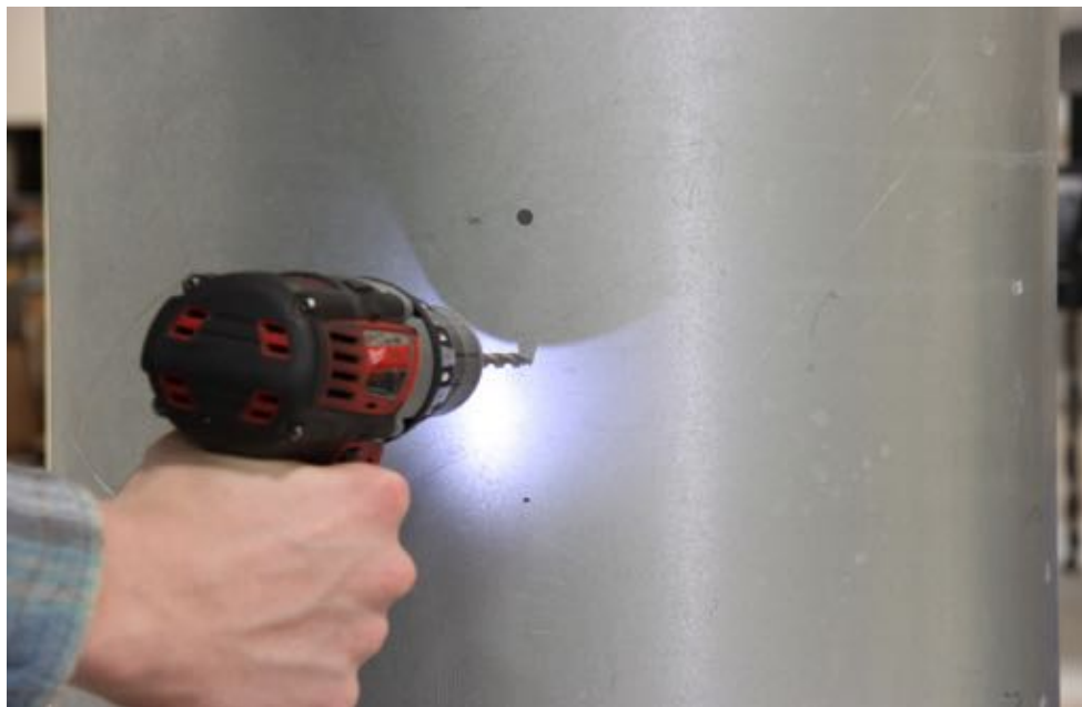
Figure 2: Drill each marked hole using the \frac{1}{4} " bit
