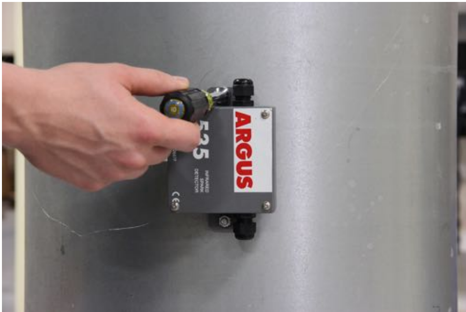
Figure 10: Place detector on bolts and tighten the nuts
